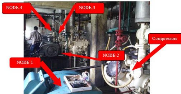
Figure 13 The experimental arrangement at refrigerator section for monitoring temperature and ammonia gas ( $NH_3$ )
