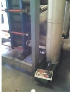
Figure 18 Photograph of the Leakage point of Ammonia gas ( $\text{NH}_3$ )
